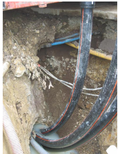
4-way duct installation drawn into drilled tunnel
