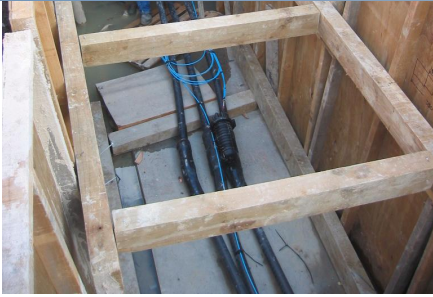
Excavation and shoring of the cable joint pits
