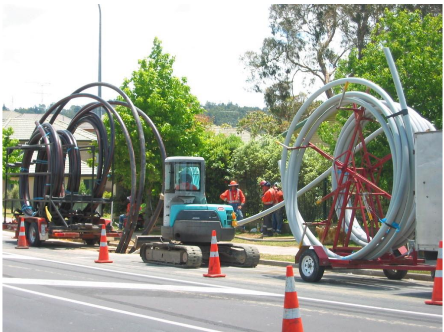
Launching the 4-way power/communication ducts into the drilled hole.
