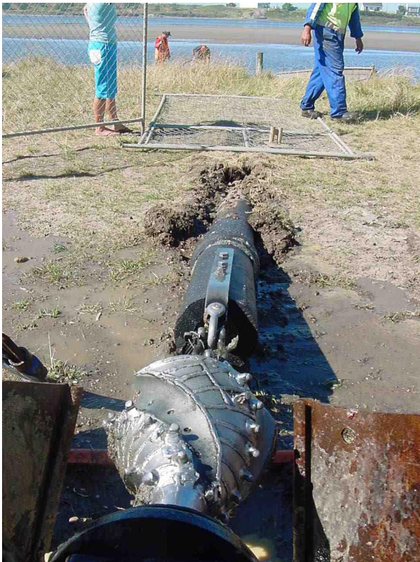
Mike Smythe (director, in his underpants) checking for drill fluid escape as the pipe is pulled up towards the drill. Ladies on the beach came down to investigate.
