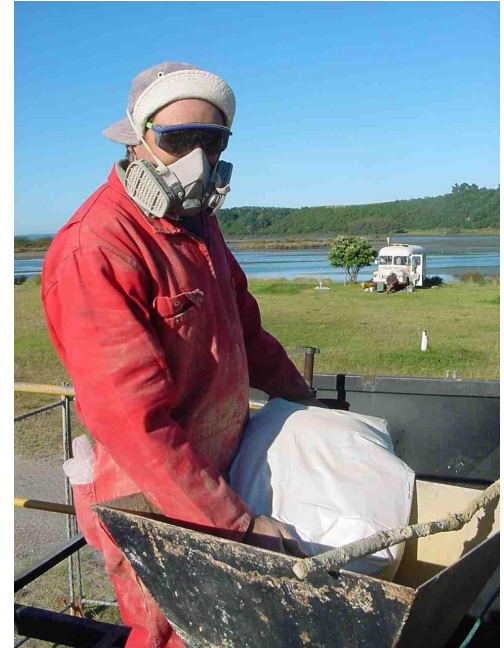
Mark Smythe adding bentonite into the hopper for mixing. All drilling fluid additives for this project were environmentally friendly
