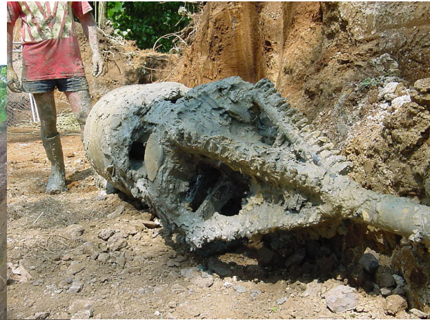
Reamer changed after encountering mud stone
