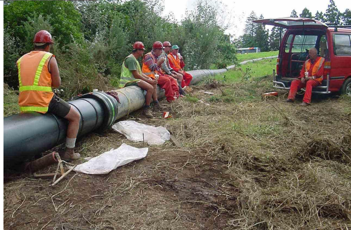
Lunch time on the day of pipe installation
