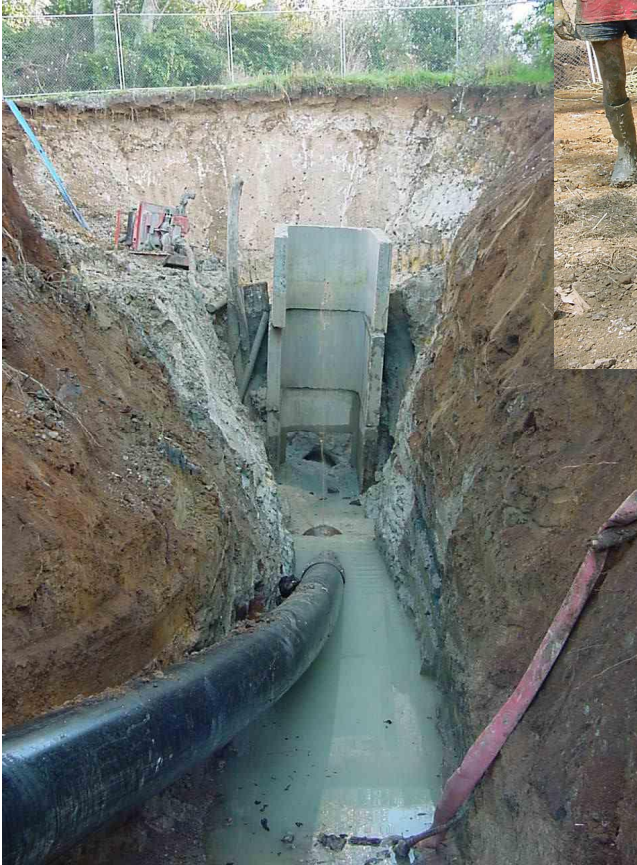
Launch pit excavation
