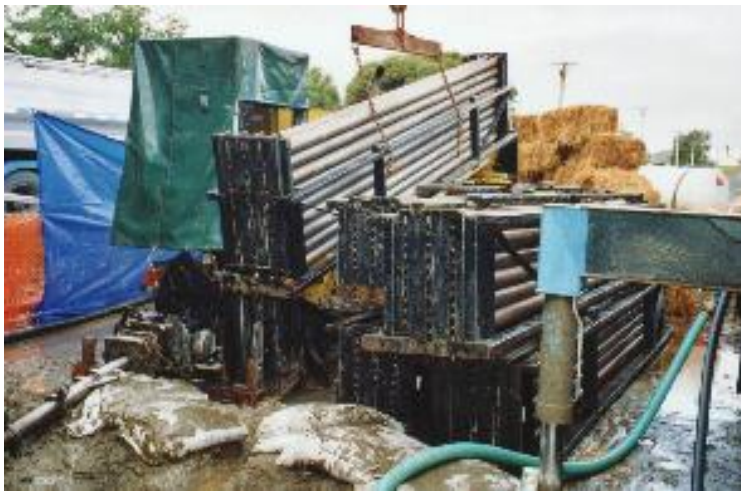
Drill with 6 racks (450m of rods)
