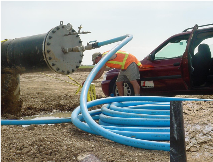
Hydraulic testing of 630Ø PE pipe
