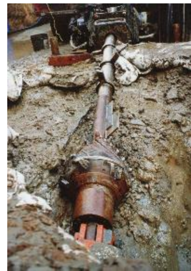
Reamer & duct arriving at the drill
