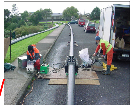
Welding and launching the pipe from Falstaff place.
