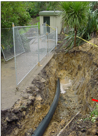
Falstaff Pump Station.
