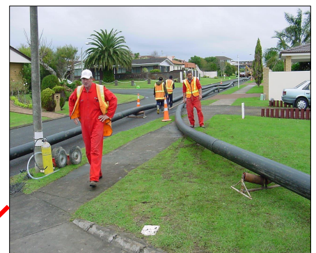
Welding and launching the pipe from Falstaff place.
