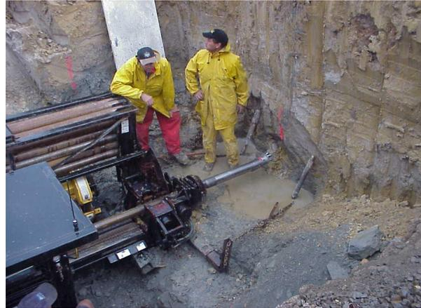
Bore path software was employed to plan this bore to calculate drilling fluid volumes, rod numbers, line, pitch and depths. This coupled with our D50x100 drill and rock drilling capacity, completed this undertaking successfully.
