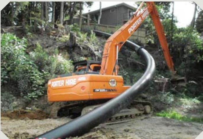
To mitigate this risk of high pullback resistance, a lot of emphasis was placed on a drill fluid (Mud Design) that both retained the hole profile and reduced friction around the pipe circumference. We estimated that 5 days were required to complete the pipe pullback, and due to good hole preparation and mud design, the pullback pressures never rose above their overnight readings.
